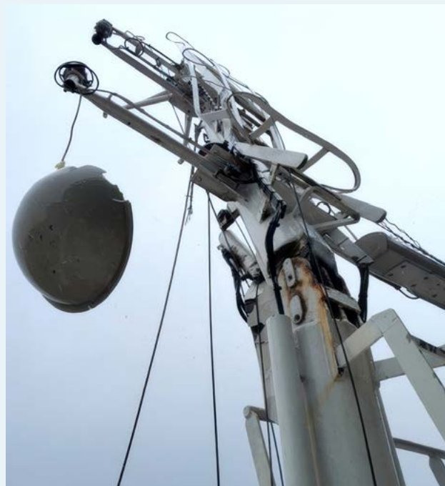
▼ Figure 26: Damage to rear mast of the Eikborg. (Source: Wagenborg)
