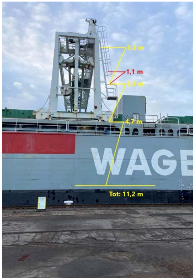
◀ Figure 11: The photo shows how the person fell down onto the quayside. Yellow lines and figures indicate the heights of the various stages of the fall. Red figures and lines mark the opening that was present between the ladder's protective cage and the railing on the narrow platform. The photo was taken on a different occasion when the draught of the vessel was different. The bottom yellow horizontal line marks the height of the quayside at the time of the accident. (Source: Statens Haverikommission)
