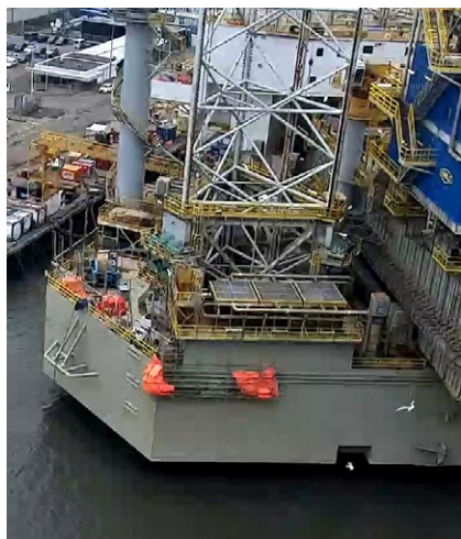
▲ Figure 15: The location of the hanging scaffold on which the welder was present. (Source: SPCM, CCTV camera 507 Lifeboat Station)
