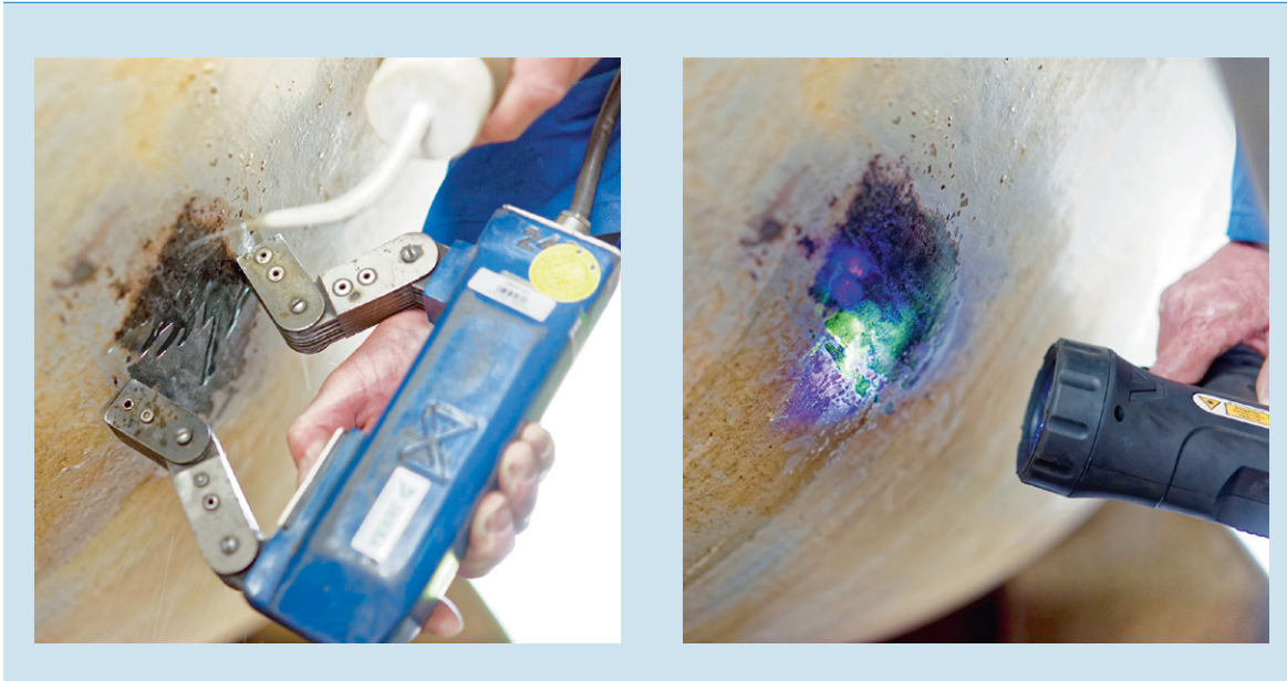
Figure 34: These photographs show the magnetic crack investigation, which was carried out at two locations on the rear wall of the tank. (Photos: Dutch Safety Board)
