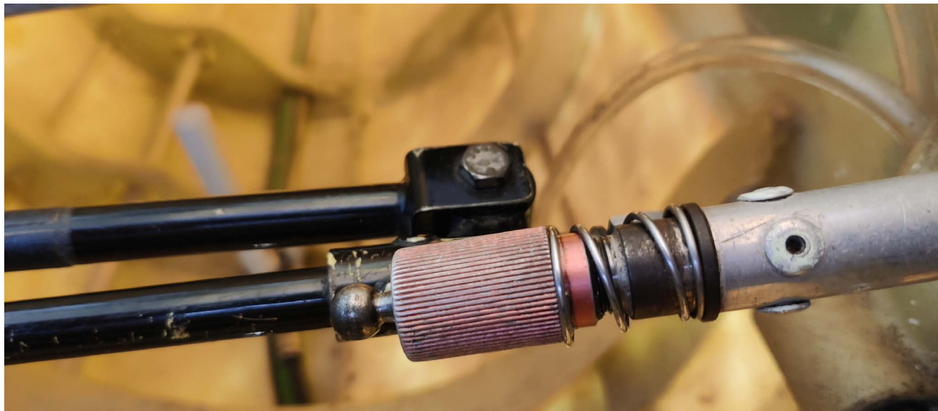
▲ The loose L'Hotellier control connection. (Source: pilot)
