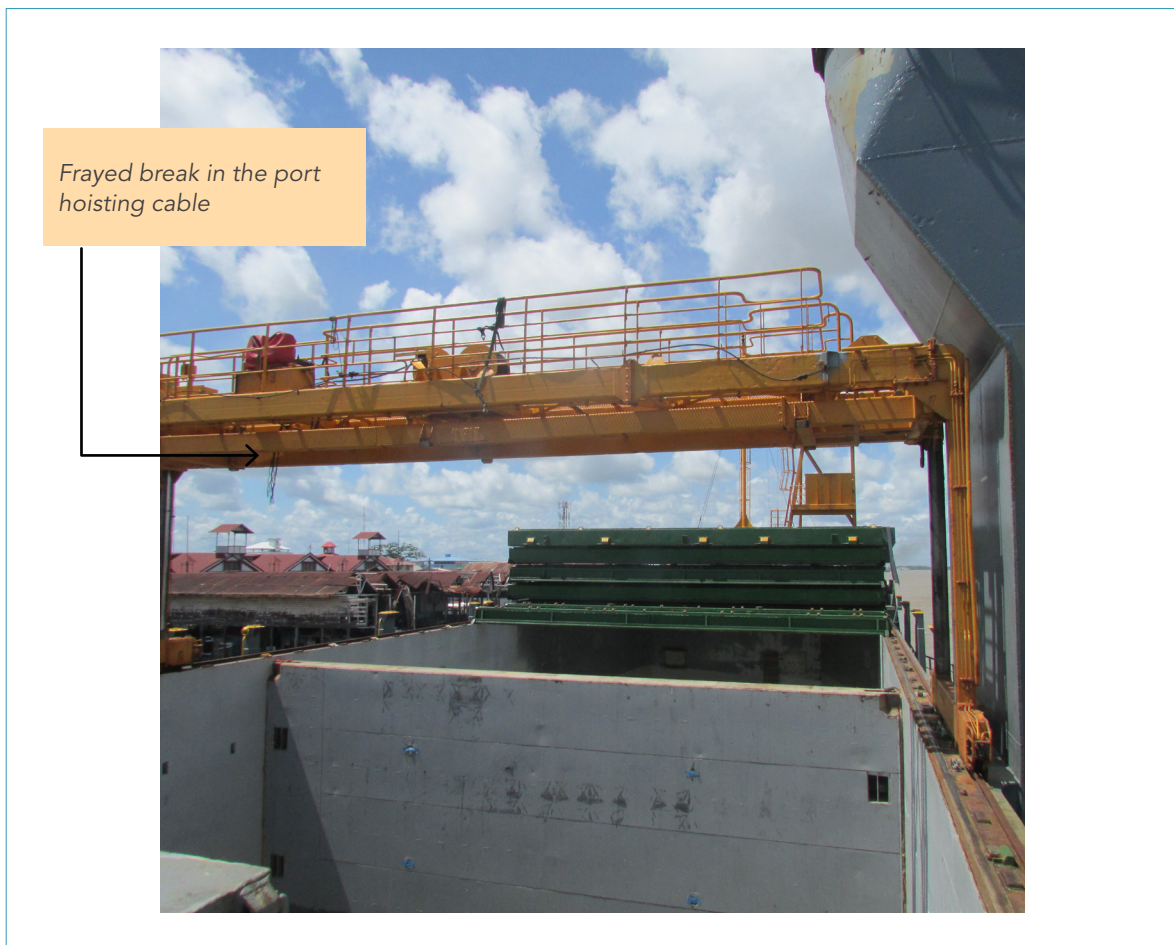
Figure 7: Hatch crane following the occurrence. (Source: ForestWave Navigation B.V.)
