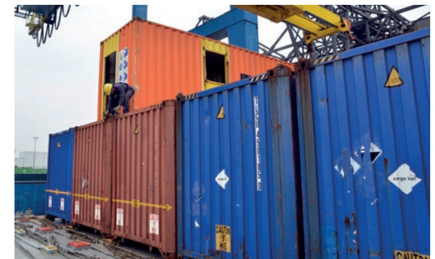
Unsafe working situation due to fall risk. (Source: Dutch Safety Board)
