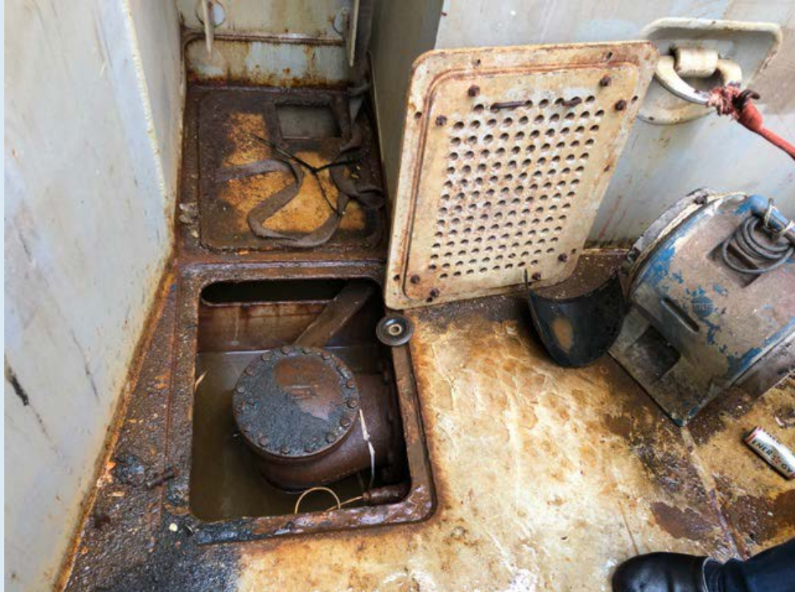
Figure 5: Bilge well in the hold of the vessel.
