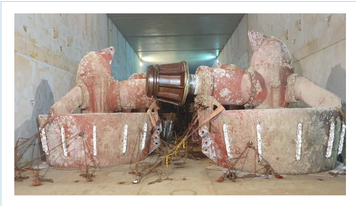
Figure 17: The thrusters on the port side and starboard side in the front part of the hold (Source: Amasus)
