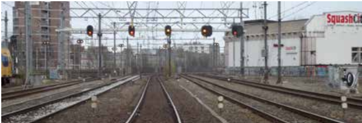
Figure 4: Signal 606 is the middle of five signals in a row and is positioned just after leaving Amsterdam Centraal station. The photograph was taken the day after the collision. Source: Dutch Safety Board
