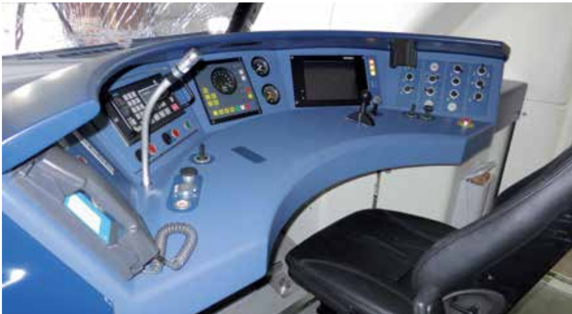
Figure 18: Top: interior of intercity's driver's compartment, at second man's station. The photo clearly shows the retracted air conditioning unit and dented rear wall, with circles around the probable contact points. Bottom: sprinter driver's compartment interior with console. Source: Dutch Safety Board
