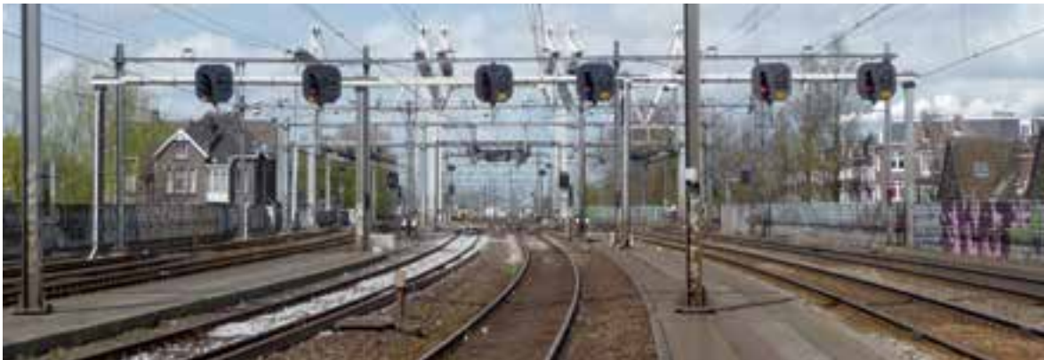
Figure 5: Signal 494 is the fourth signal from the left and is positioned just before the Singelgracht bridge. The photograph was taken the day after the collision; the sprinter had been towed away by this time. Source: Dutch Safety Board
