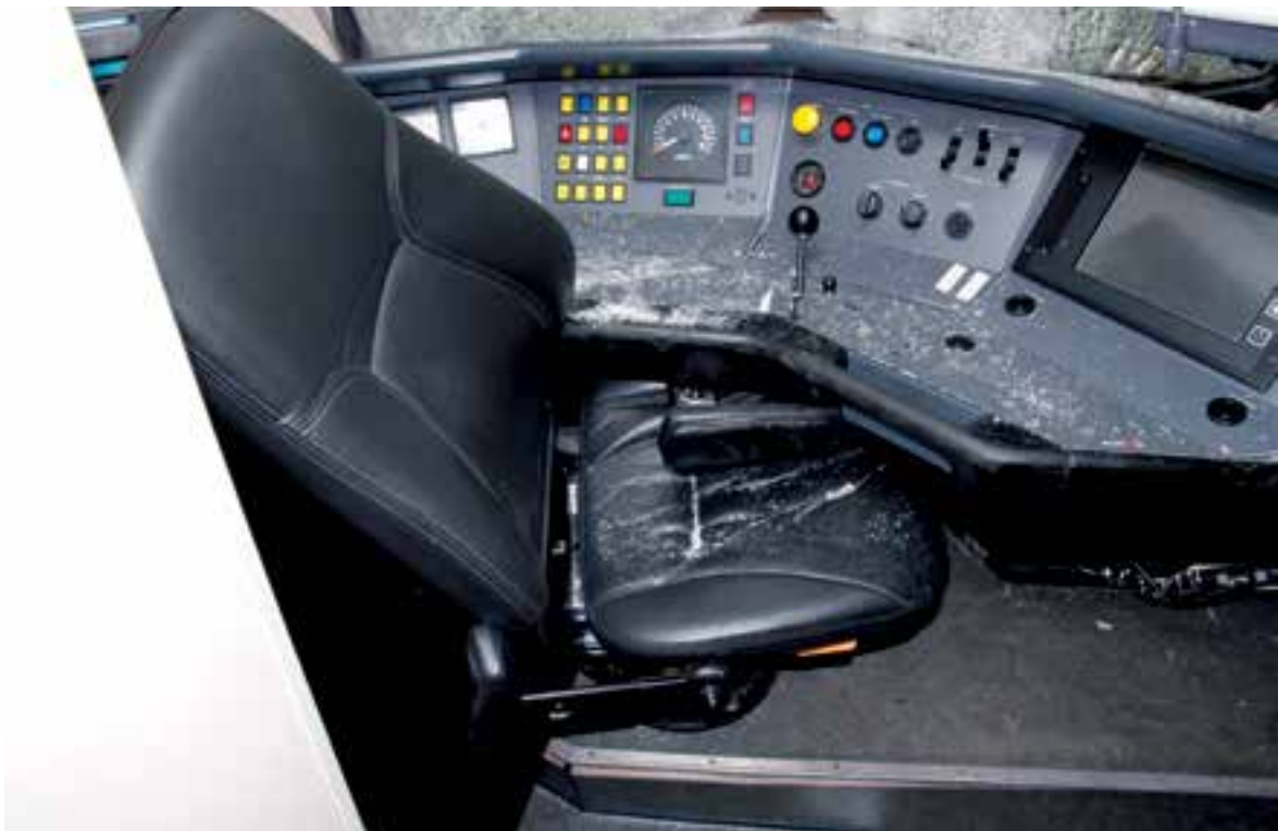
Figure 9: Upper left: damaged nose of the intercity. Upper right: the air conditioning unit that had been pushed backwards. Bottom: damage to the driver's desk. Source: Dutch Safety Board
