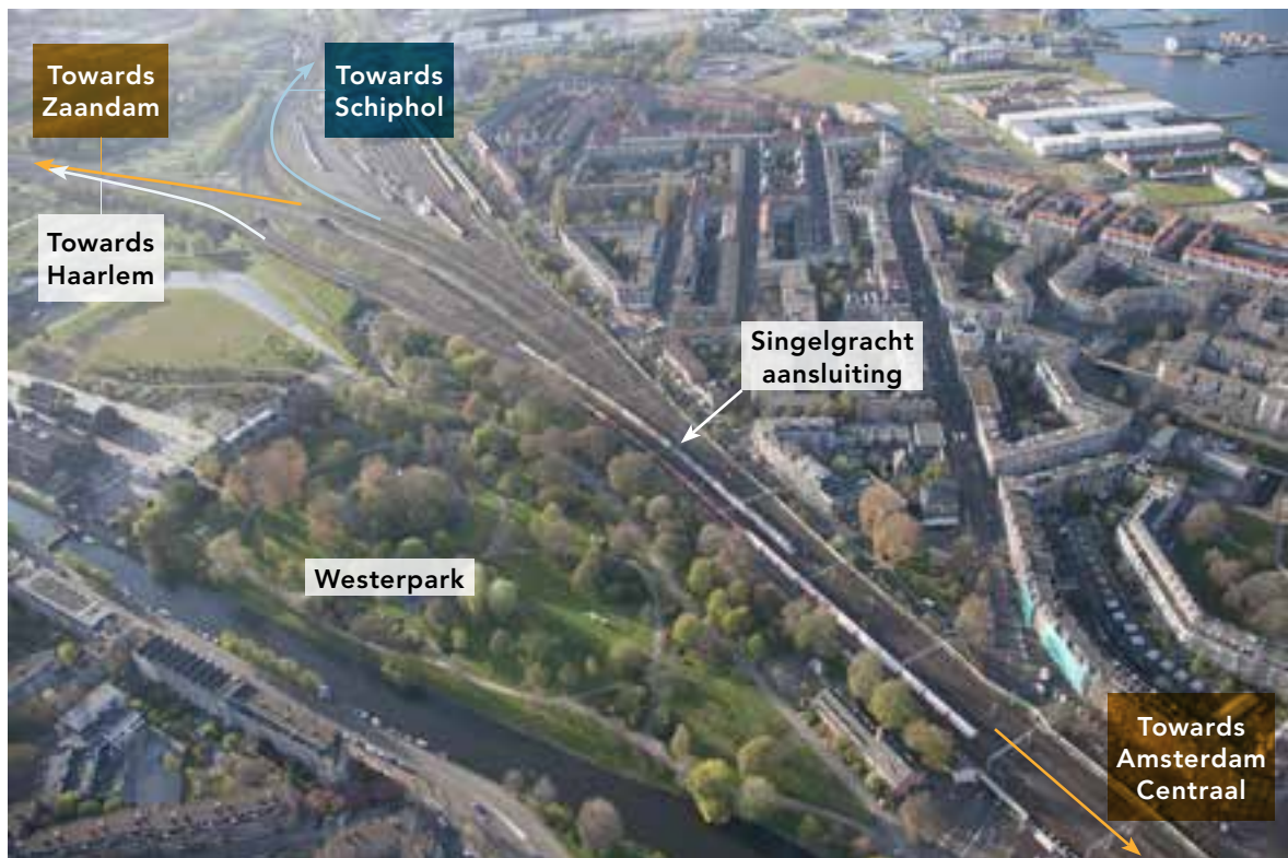
Figure 2: Aerial photograph of the accident site. Source: KLPD.
