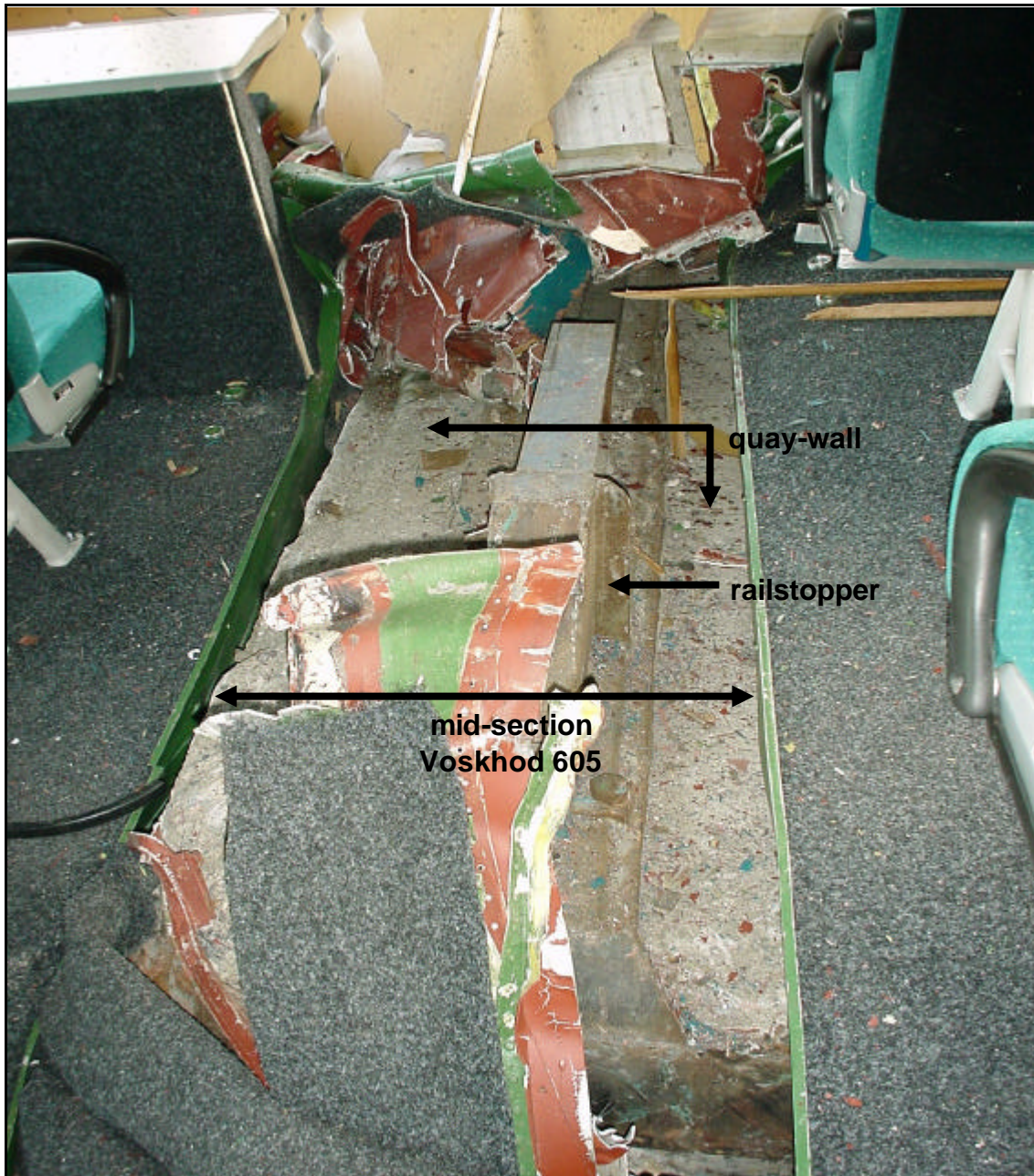
Figure 3: Photo of the quay wall and a rail that have torn open the mid-section, taken from the front passenger compartment of the Voskhod 605.
