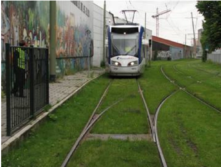
Figure 12- Vehicle approaching an openable switch
