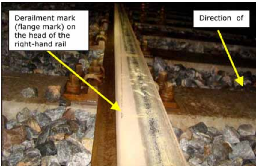
Figure 12: This photo shows the derailment marks on the head of the right-hand rail.
