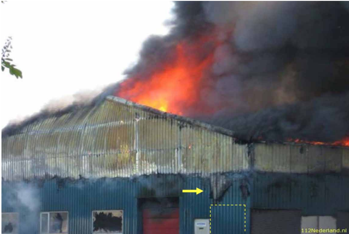
Photograph 4 Back of the shed when the fire was fully ablaze. The yellow arrow is pointing to the 'V' pattern on the outside wall. The yellow dotted line indicates the outline of the meter cupboard located on the other side of the wall.
