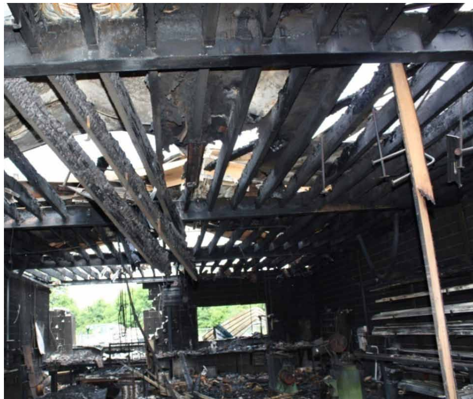
Photograph 5 Aluminium workshop – thermal attack from attic to workshop
