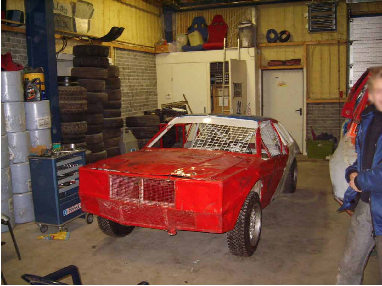
Photograph 3 The inside of the storeroom. On the left-hand side at the back, with the door open, is the meter cupboard where the fire started. The yellowish coating on the higher parts of the walls is exposed polyurethane foam.
