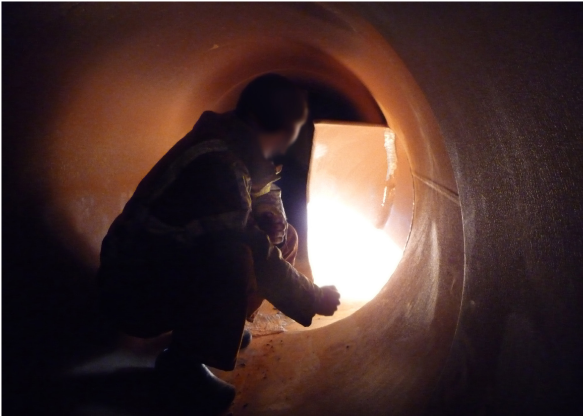
Figure 2: Inside of the loading pipe, during welding.
