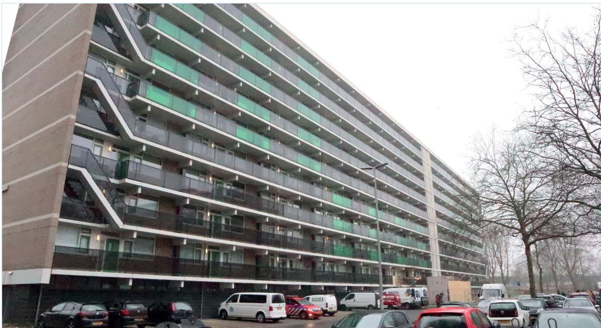
Figure 1: Block of flats where the fire raged on New Year's Day 2020. (Source: Dutch Safety Board)
