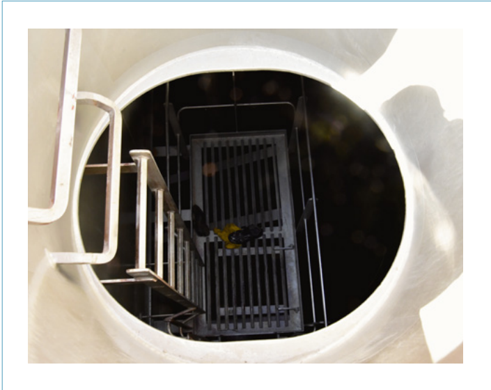
Figure 2: Top view of tank with view of the first platform.
