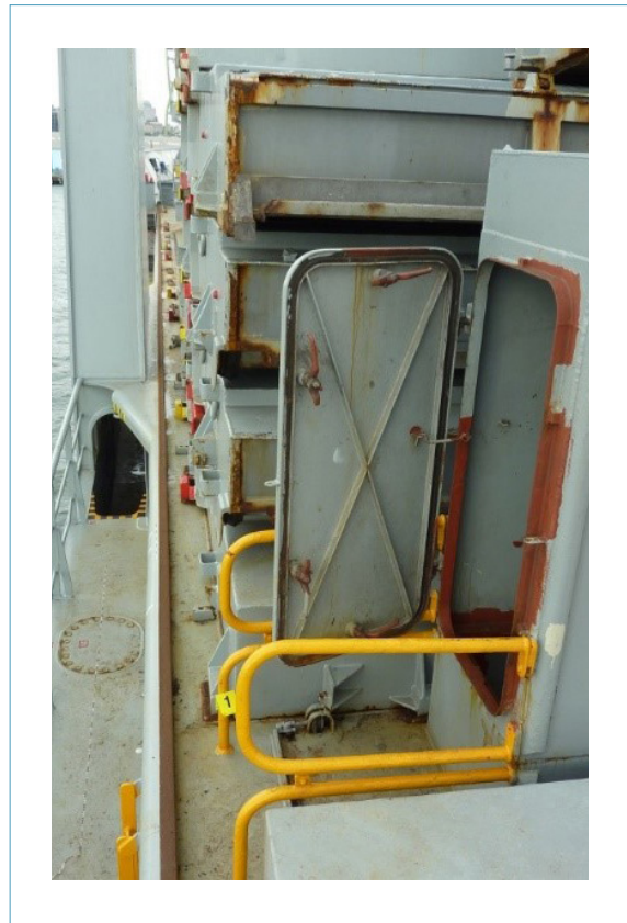
Figure 4: Hold entrance on port side, showing the watertight door and the stacked hatches.
