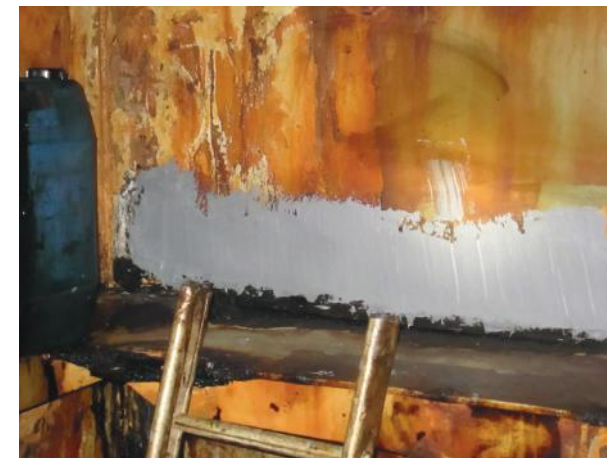
Repair with epoxy resin. (Photo: Iver Ships)
