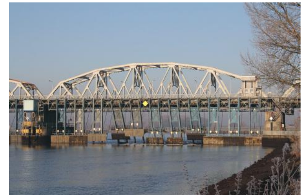
The weir at Grave.
