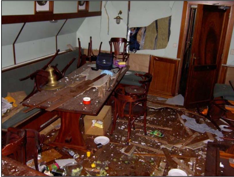
Figure 7: Damage to the interior on the port side, view towards the bow of the ship (photo: Dutch Safety Board)
