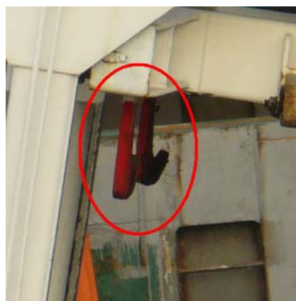
Photo 7: Enlargement of bent hooks.
