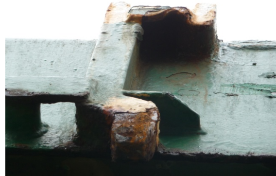
Photo 9: Damaged attachment point of the fallen hatch.
