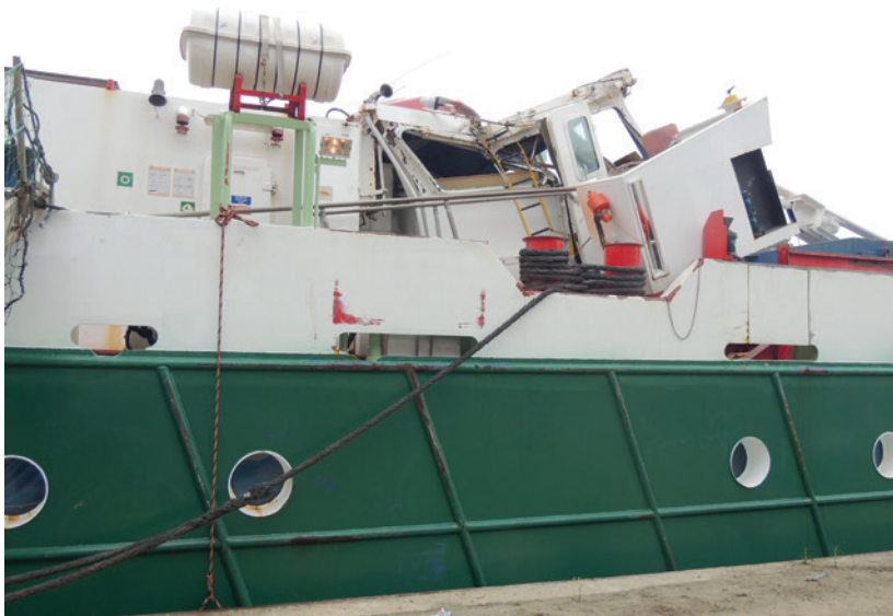
Left and right the damage to the wheelhouse of the Amadeus Amethyst.
