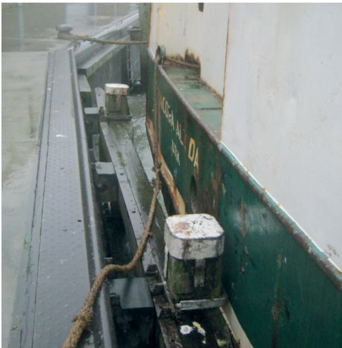
Figure 2: Wooden fender wall and stern of the UK268 Jacoba Alyda. (Source: Inspection SZW-direction Arbo)
