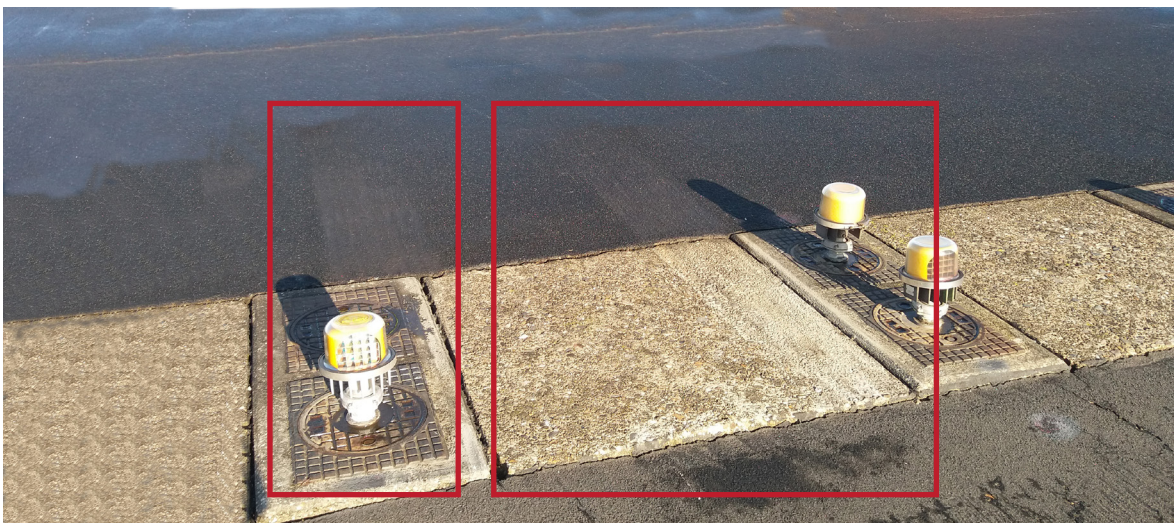
Figure 1: Traces of the main landing gear (marked with a red frame) visible on the runway edge after the occurrence. The three damaged lights had already been replaced. (Photo: Amsterdam Airport Schiphol)
