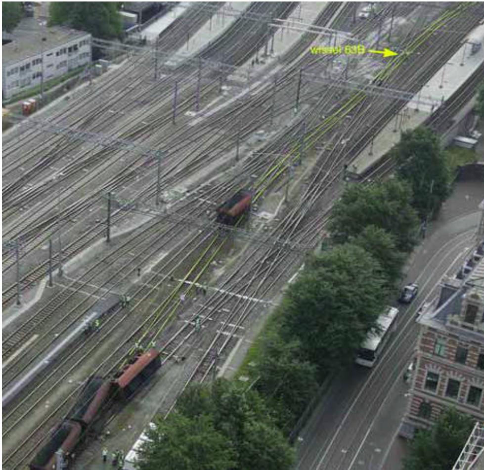
Illustration 2 Defective set of points 63, track and final position of the derailed wagons
