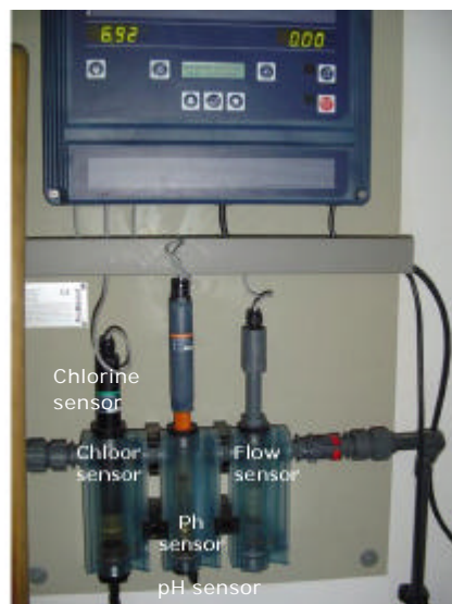
Illustration 6. The measuring plate with sensors
