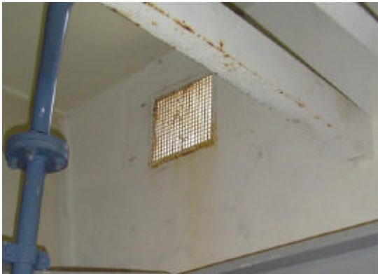
Illustration 8a. A ventilation grate
