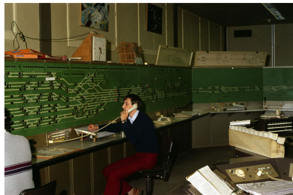
Figure 9 Amsterdam Train traffic control post pre 1995. For each train, a route was set by hand. The advantage of this process was that in the event of disruptions, the train traffic controller could set any conceivable route. All this information was brought together on the panel in front of him. The train traffic controller saw the local problems on the panel, alongside all possibilities for solving those problems.
