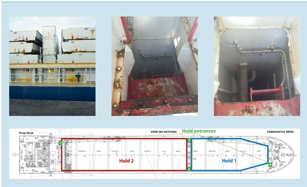
Figure 1: Below: ship's configuration. Top left: access to hold amidships via portal. Top middle and right: View looking down ladders from portal and platform above ladders. (Photo: Dutch Safety Board)
