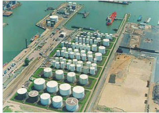
Fig. 4 The Vopak Terminal TRR storage facility for chemical substances in Botlek, Rotterdam. Left, in the open air, is the filling station for tank wagons.
