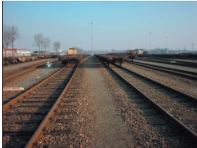
Fig.3. The Waalhaven marshalling yard, looking east.
