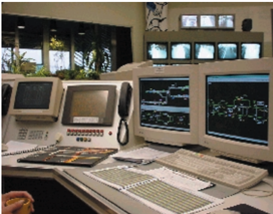
Fig. 2 Traffic controllers post. The two computer screens provide a schematic overview of the network and the positions of the metros and high-speed trams on the network. Using the keyboard, routes are selected. The adjacent system provides the link to the drivers on lines 53, 54 and the emergency services. The next piece of equipment provides a link to the drivers on line 51 (high-speed tram). To the left, outside this picture, is the installation for the station PA system. In the background, the monitors which provide a view of the stations, are just visible.
