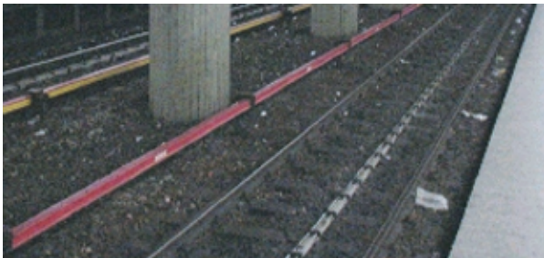
Fig. 3. The ballast bed and tracks. The red construction is the electrical power supply which first has to be short-circuited, before walking on the ballast bed, or extinguishing with water.
