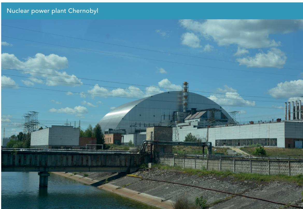
Figure 3: Photograph of the Chernobyl nuclear power plant in 2017, which shows the steel arch that covers the destroyed reactor. (Source: Dutch Safety Board)
