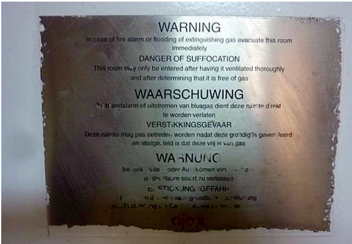
Figure 4: Warning on the access doors to the stairwell. (Source: Ameyde Marine)
