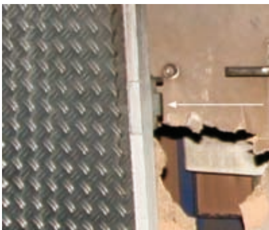
Figure 6: Bolt on the door to cell 5 turned outwards
