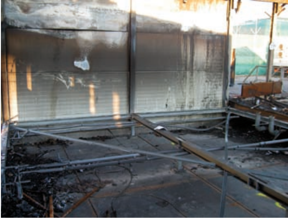
Figure 11: Far wall on the inside, where cell 11 was situated. The cell has been removed in this picture. To the left of the centre of the picture, the intense burn imprint, which formed next to the bunk bed in the cell, is visible.
